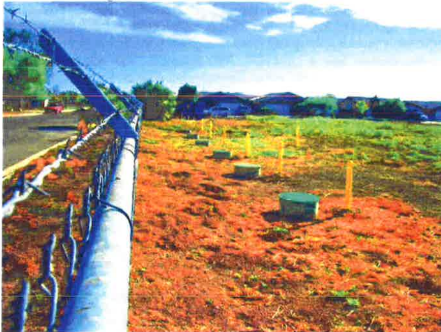
Existing wastewater facility with leach field, looking south on Poe Colonia Road
