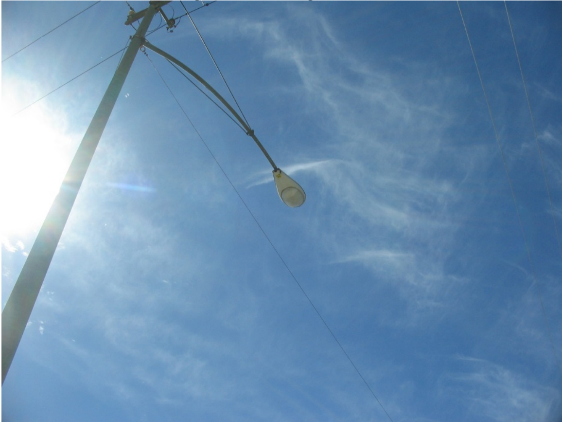
Existing streetlight located on Highway 111
